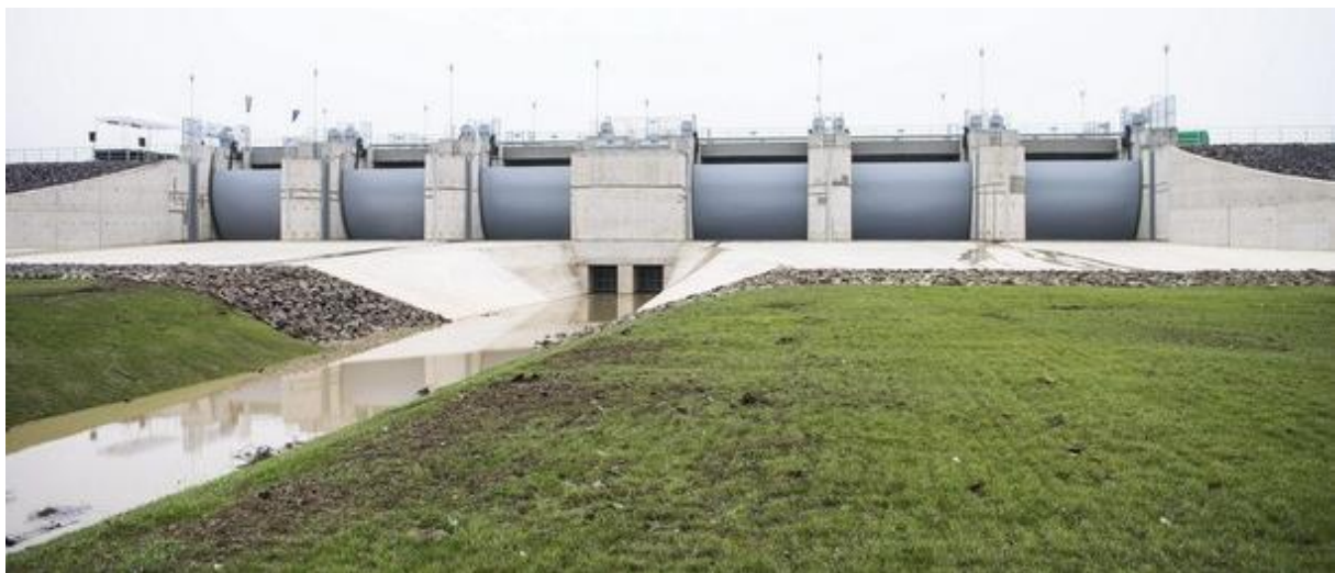
Figure 4.23: The Beregi tidal reservoir's inlet structure, consisting of 6 segmental panels, between Tarpa and Tivadar Source: MTI/Balázs Attila
